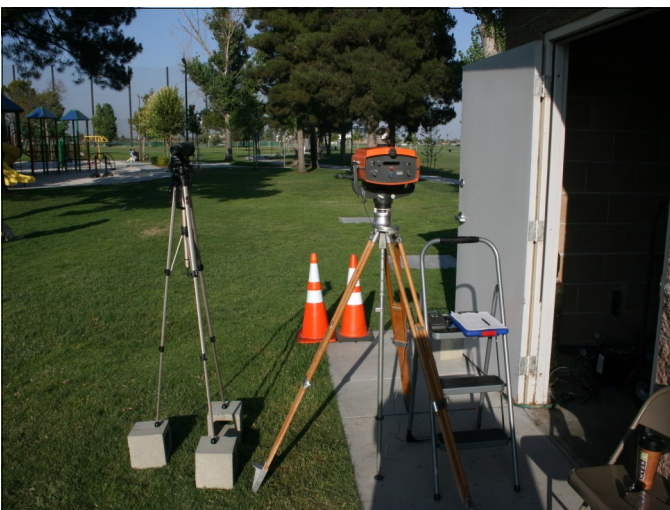
MZ-1 Monument Construction & Surveying
