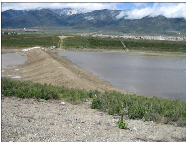
New San Sevaine Basin No. 5 Conservation Berm
